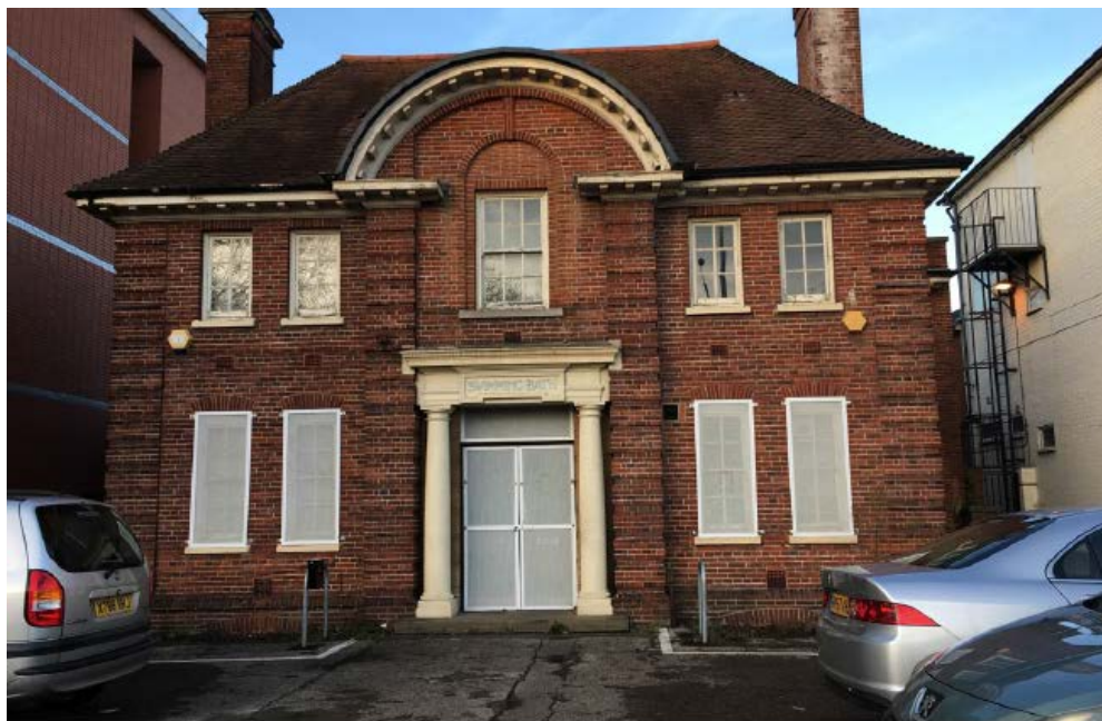
Figure 14.1: Arthur Hill Pool, Kings Road frontage (source of image: Savills)
