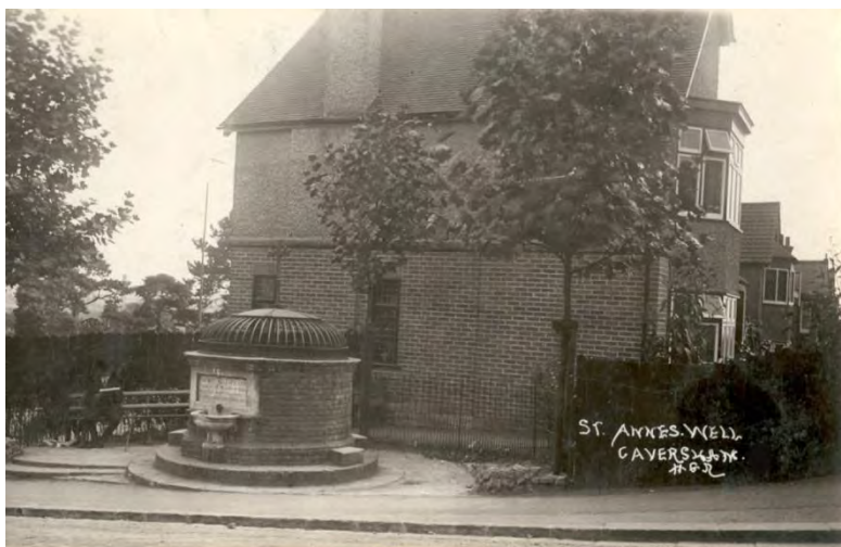
Figure 6.6 St Anne's Well and surroundings circa 1930 (Copyright. Image reproduced courtesy of Reading Library Collection).
