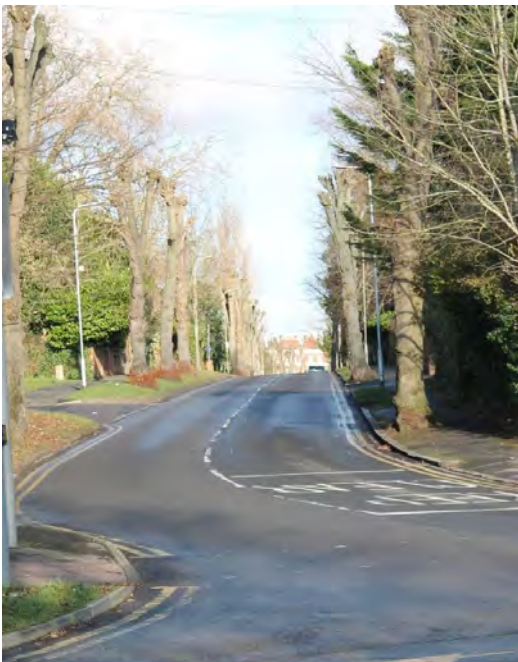
Figure 9.3 View towards Bath Rd and the Conservation Area from the Berkeley Avenue junction
