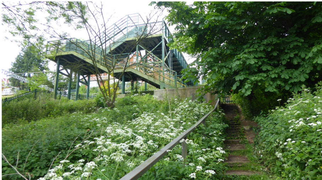
70 steps down from footbridge over railway to Thames. Cyclists would have to carry bicycles up or down these steps.
