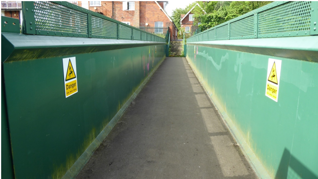
Footbridge over railway to rear of former Roebuck Inn showing 11 steps down onto bridge. Bridge width 2.2 metres.
