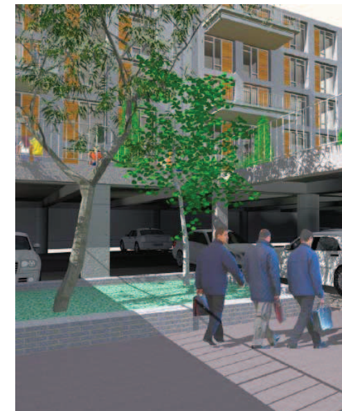
Figure 11.5 Light wells allow natural lighting and ventilation into lower level parking areas.
