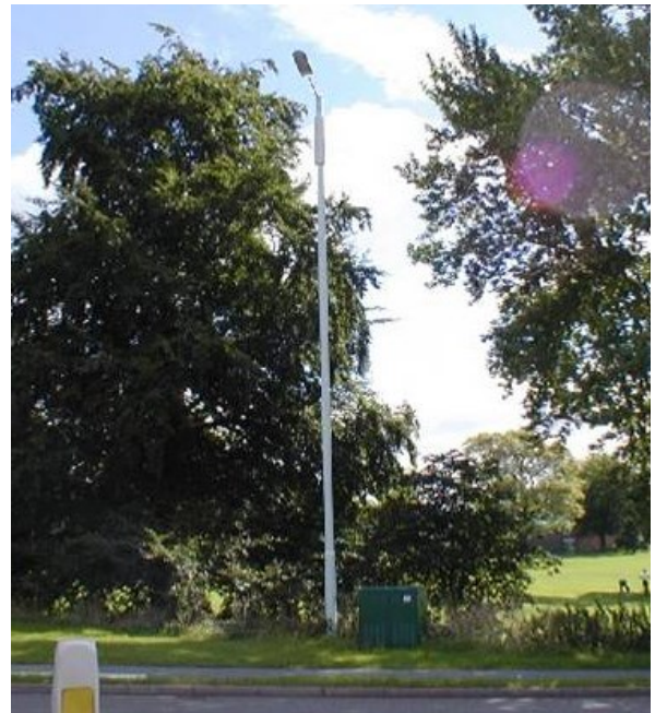
Figure 6: Example of lamp column ‘swap-out’ - with antenna shroud below street lamp and ancillary green equipment cabinet.
