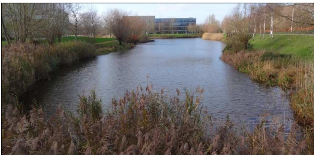
Figure 7.1: View West across Longwater Flood Relief Channel at Green Park
