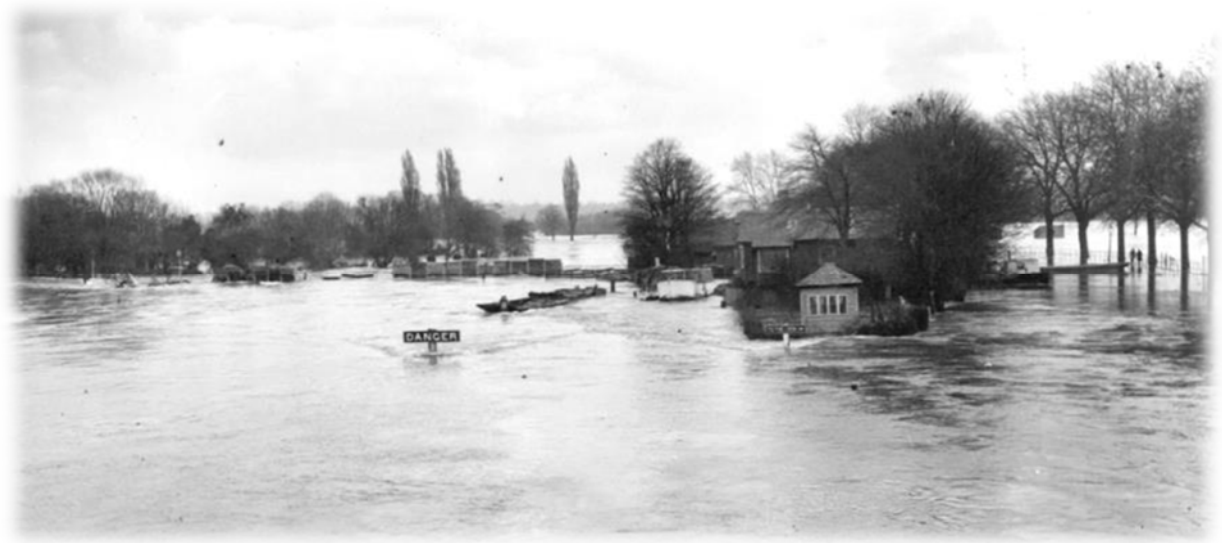
Figure 8.3: River Thames - View towards Caversham Lock and Weir in 1947 Flood Event
