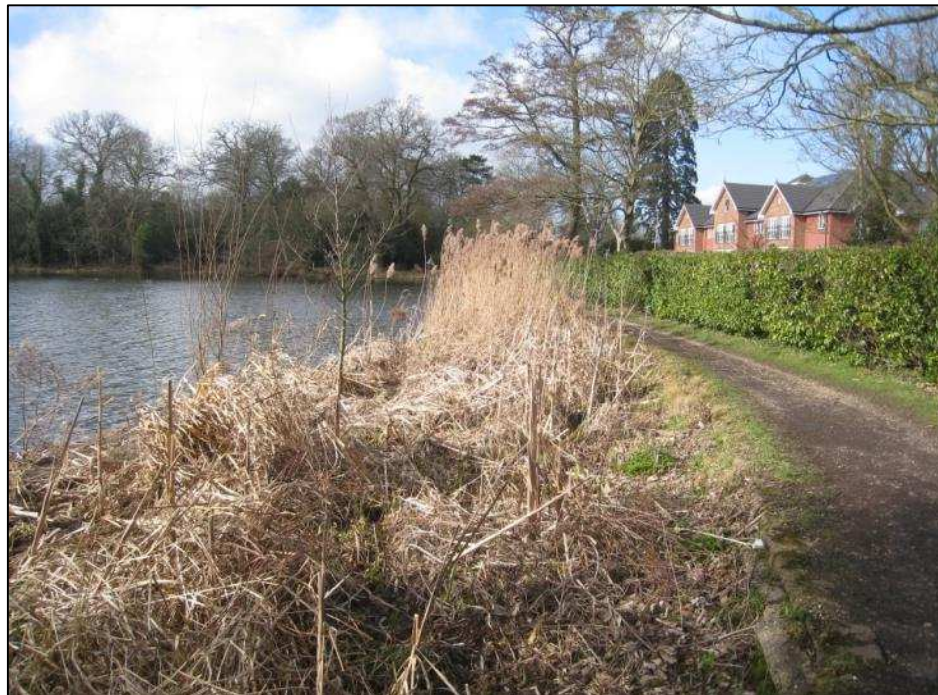
Figure 6.11: Whiteknights Lane – View along Embankment Dam
