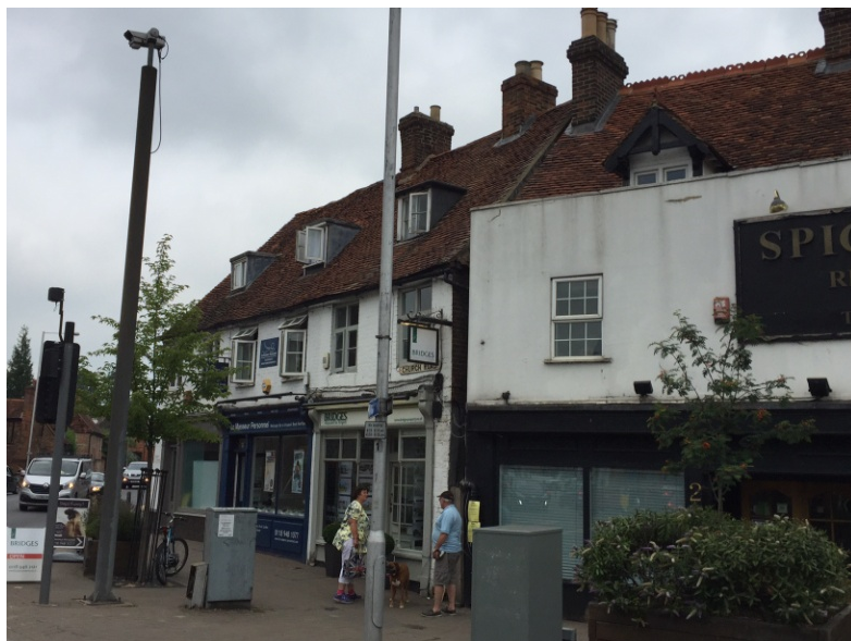
UPVC window replacements in a listed building. Opportunities should be sought to reverse such damage when maintenance, replacement or alterations are carried out. In the foreground a utilitarian mast, pole and cabinets also detract.
