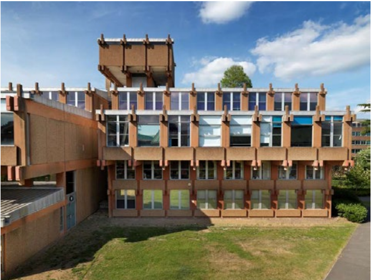
Figure 19. View of Grade II Listed URS Building
