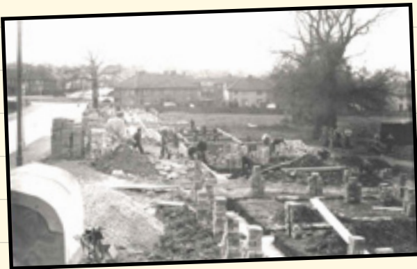
The building of the Shinfield Road Council housing estate 1924. Materials were moved by horse and cart and by a steam traction engine. 1920-1929
