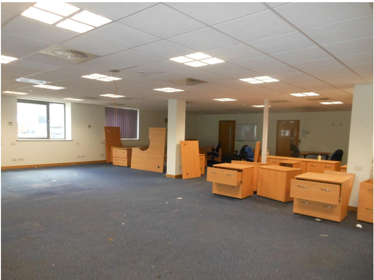
Interior of Rear Building
