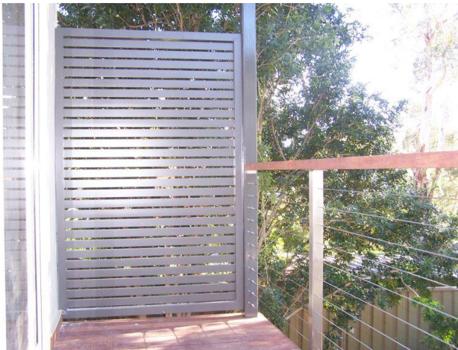
Figure 63 Examples of balcony mitigation – Side Screen
