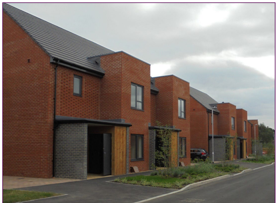
Figure 6: Local authority new build homes at Conwy Close
