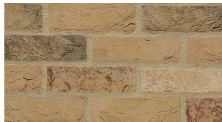
Main Facing Materials
