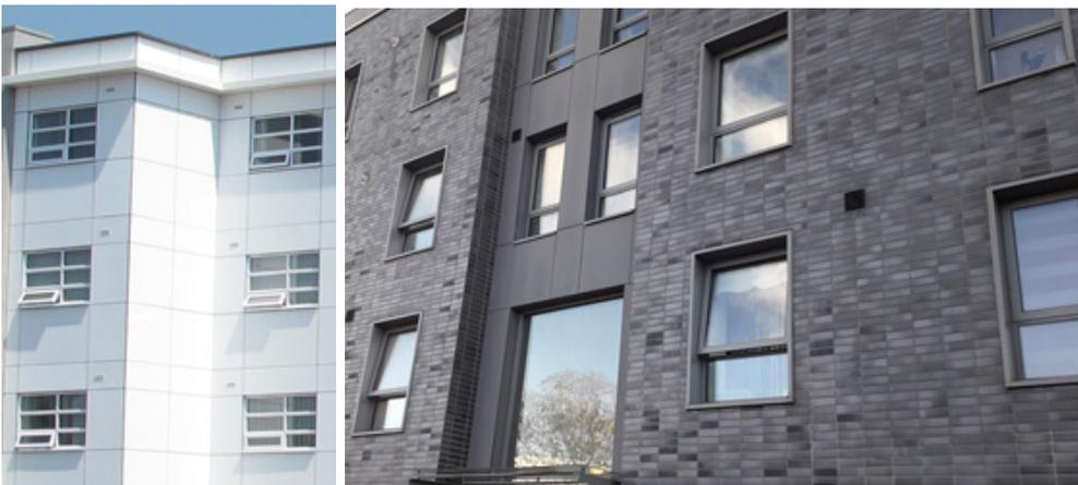
Figure #14-1: Examples of restricted window openings; (left): Only one of six panes was openable, and only to a limited extent - the flats overheated ([GHA Preventing overheating report, 2014](#)); right: only the top 2/3 part of windows opens, and the opening is restricted to only a very small gap.
