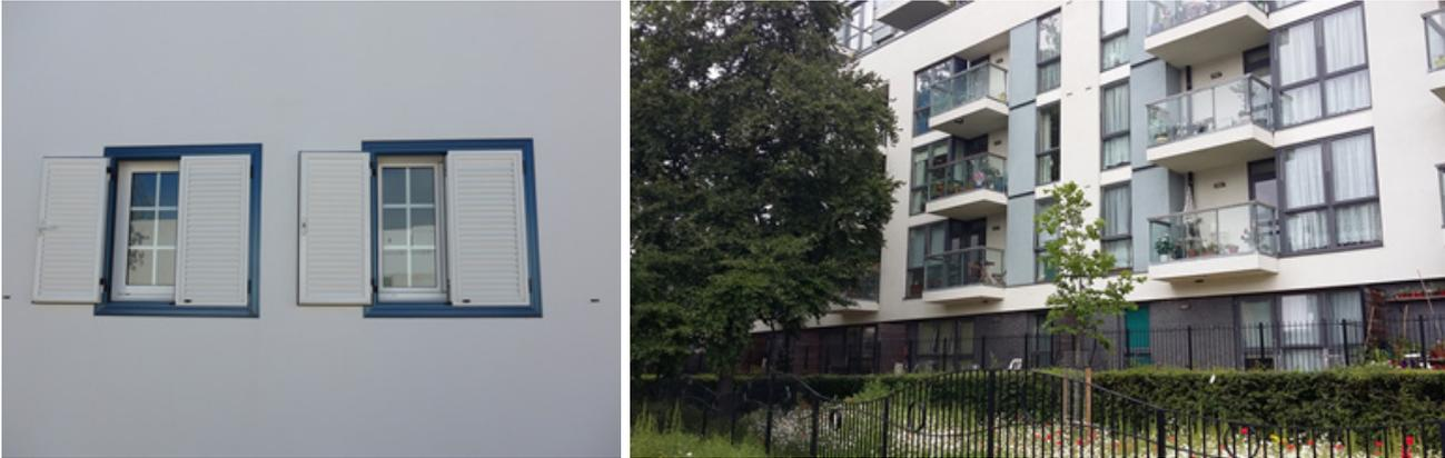
Figure 9-1: Examples of light-coloured (high albedo) facades, likely to be of lower temperatures than surfaces such as brick.
