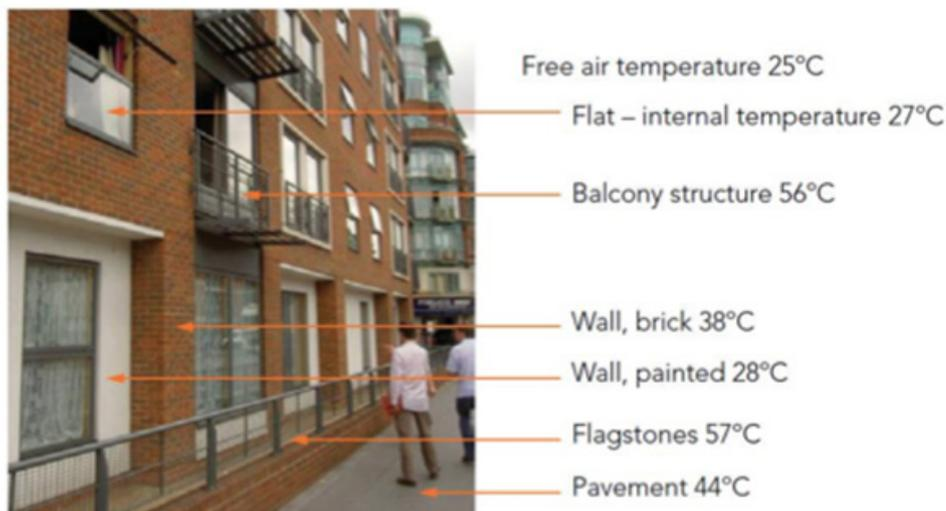
Figure 9-1: A study carried out by the BRE showed that surface temperatures contributed to overheating risk, with south-facing exposed brick facades and tarmac areas nearby contributing to high temperatures near air inlets.
