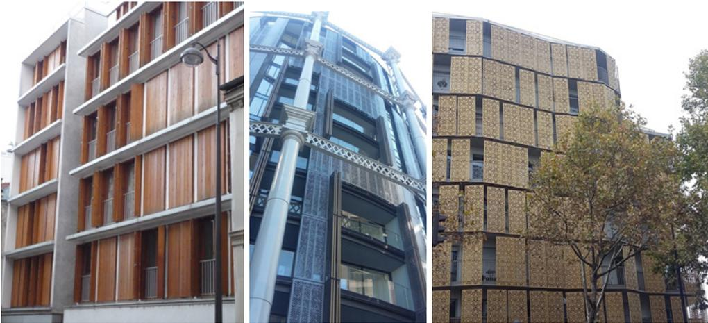
Figure #13-1: Examples of movable shading devices. They are used differently across the facade, showing user adaptation.
