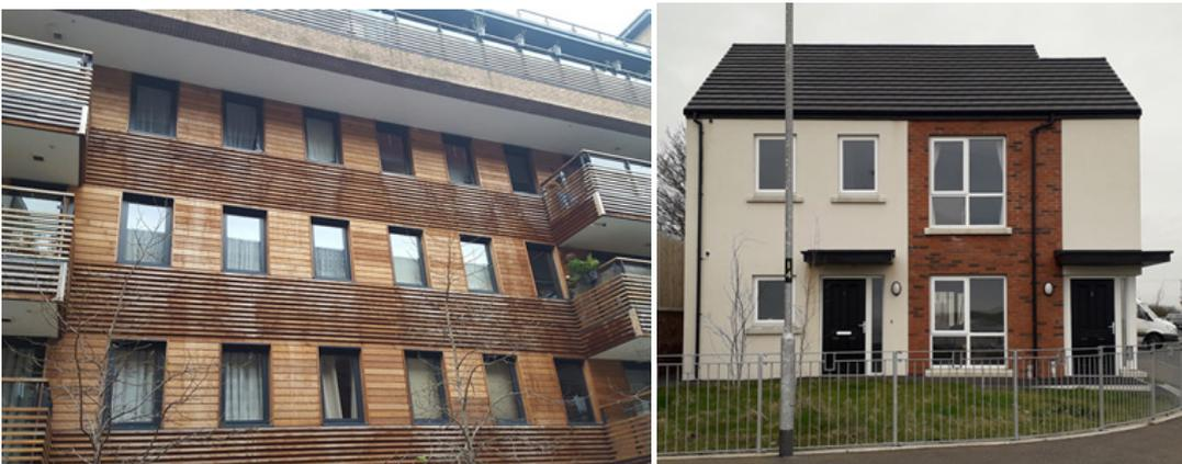
Figure #6-2: Example of glazing proportion between 35% and 50% of facade area
