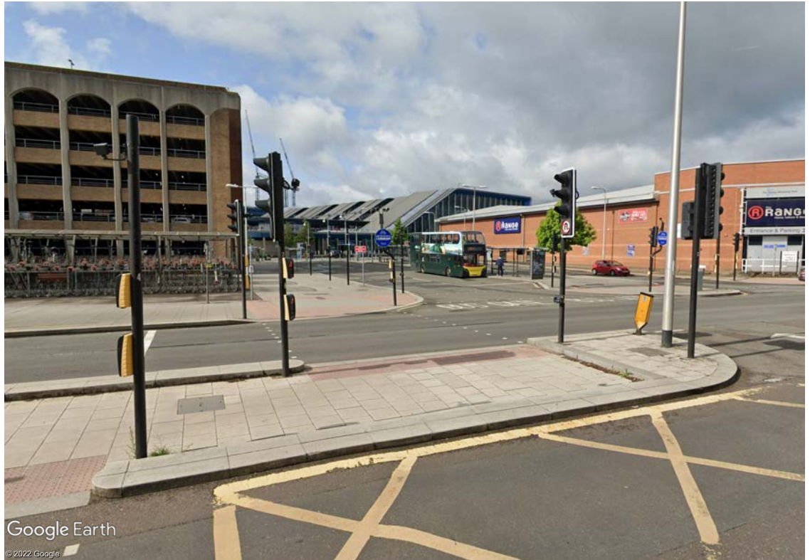
Figure 18. The station is already a highly legible landmark in views from Vastern Road
