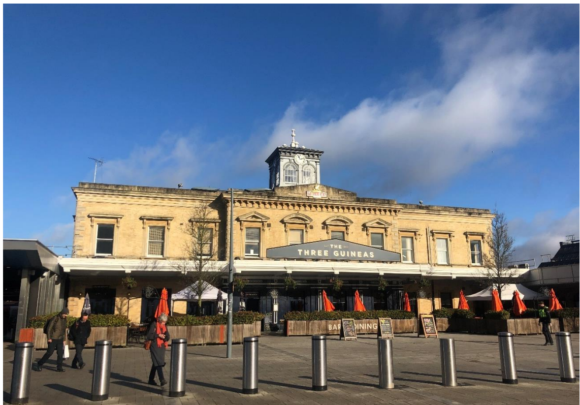
Figure 3.2 Main Building of Reading General Station
