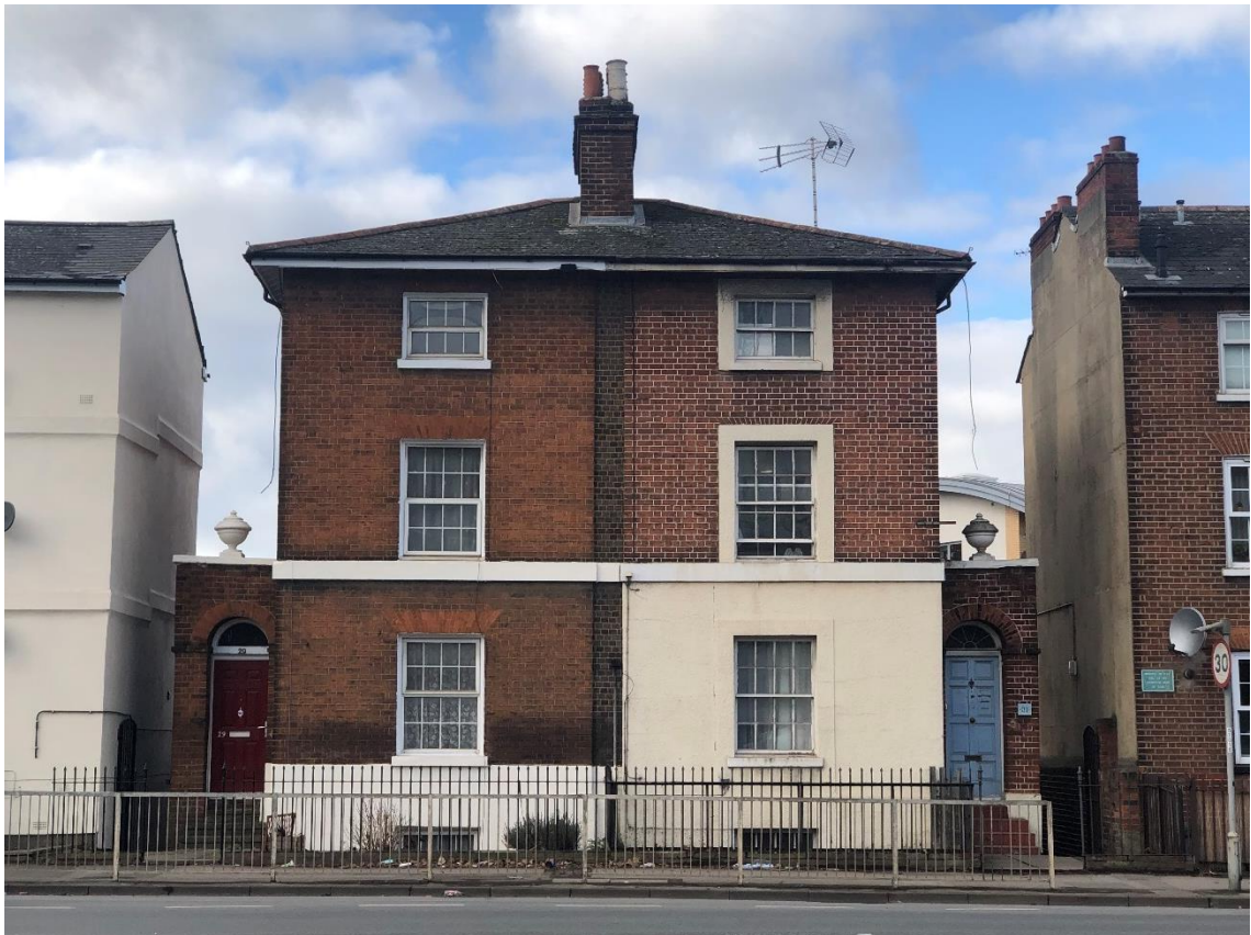
Figure 3.9 29 and 31, Caversham Road
