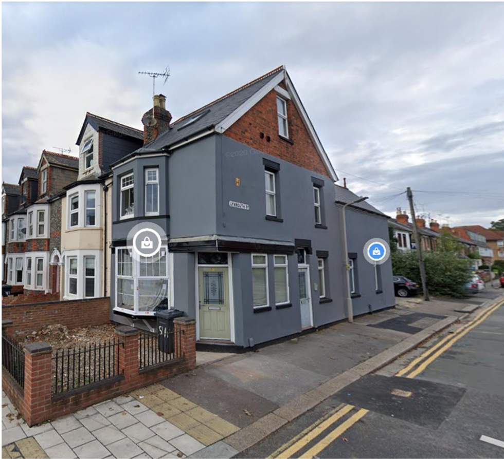
Figure 9. 51 Vastern Road (photo from Google Streetview).
