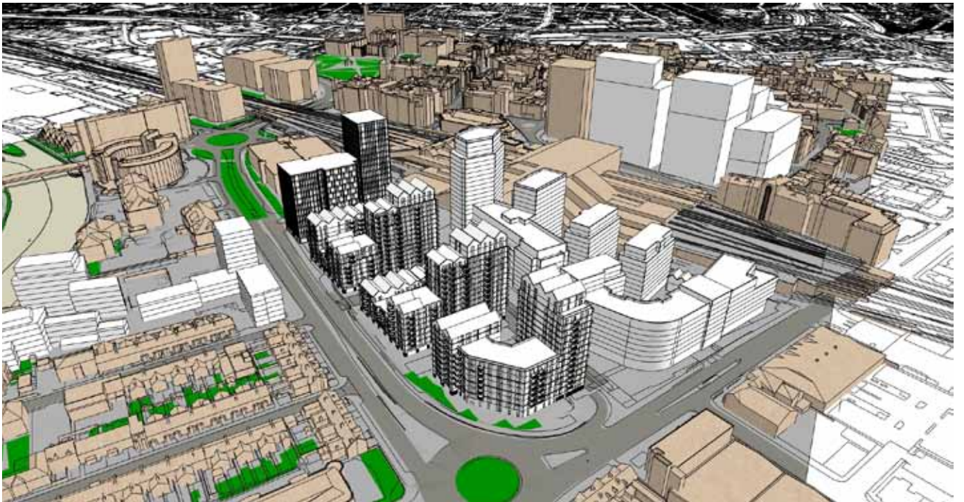
Figure 6. Aerial view showing the consented schemes for Royal Mail and SSE plus Illustrative Scheme on appeal site.
