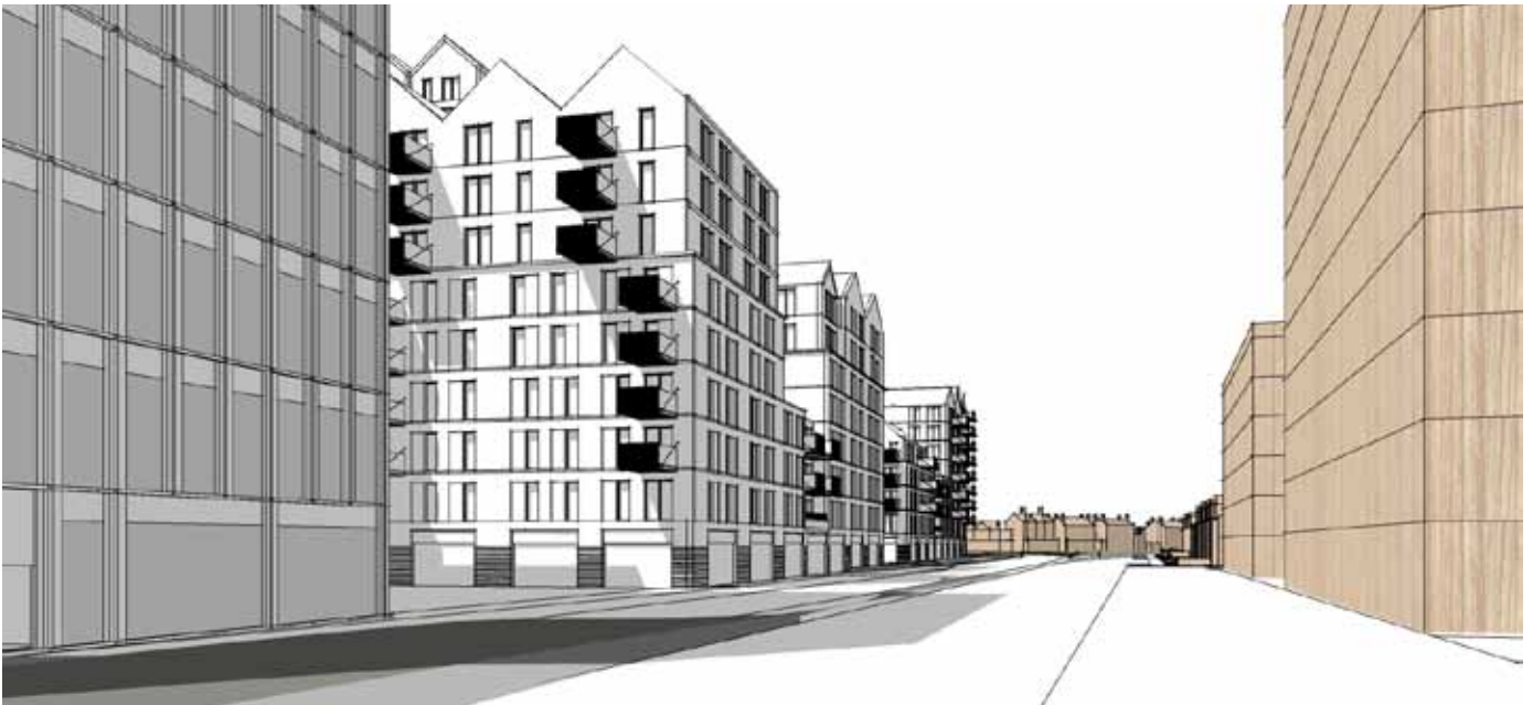
Figure 5b - View along Vastern road looking North-West towards the Aviva site
