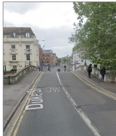
VIEW TOWARDS SOUTH
