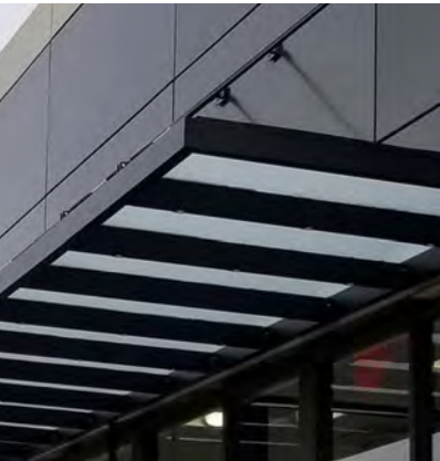
PROPRIETARY GLASS CANOPY ABOVE ENTRANCE DOORS
