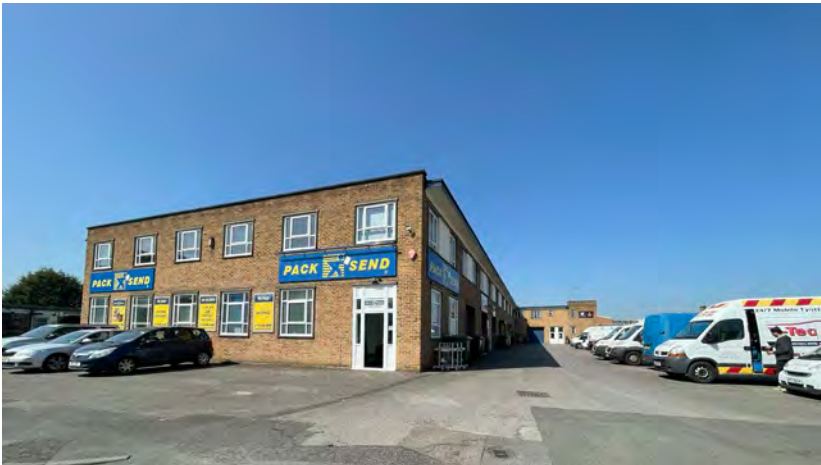
12: EXISTING EMPLOYMENT BUILDING ALONG MILFORD ROAD
