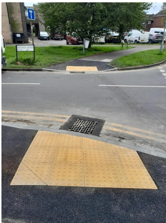
Figure 4.1: Dropped kerb at the junction of Hexham Road and Corbridge Road
