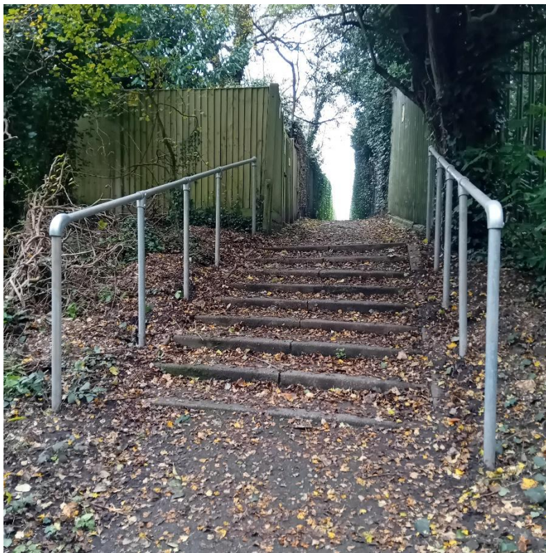
Figure 4.2: New pedestrian handrail
