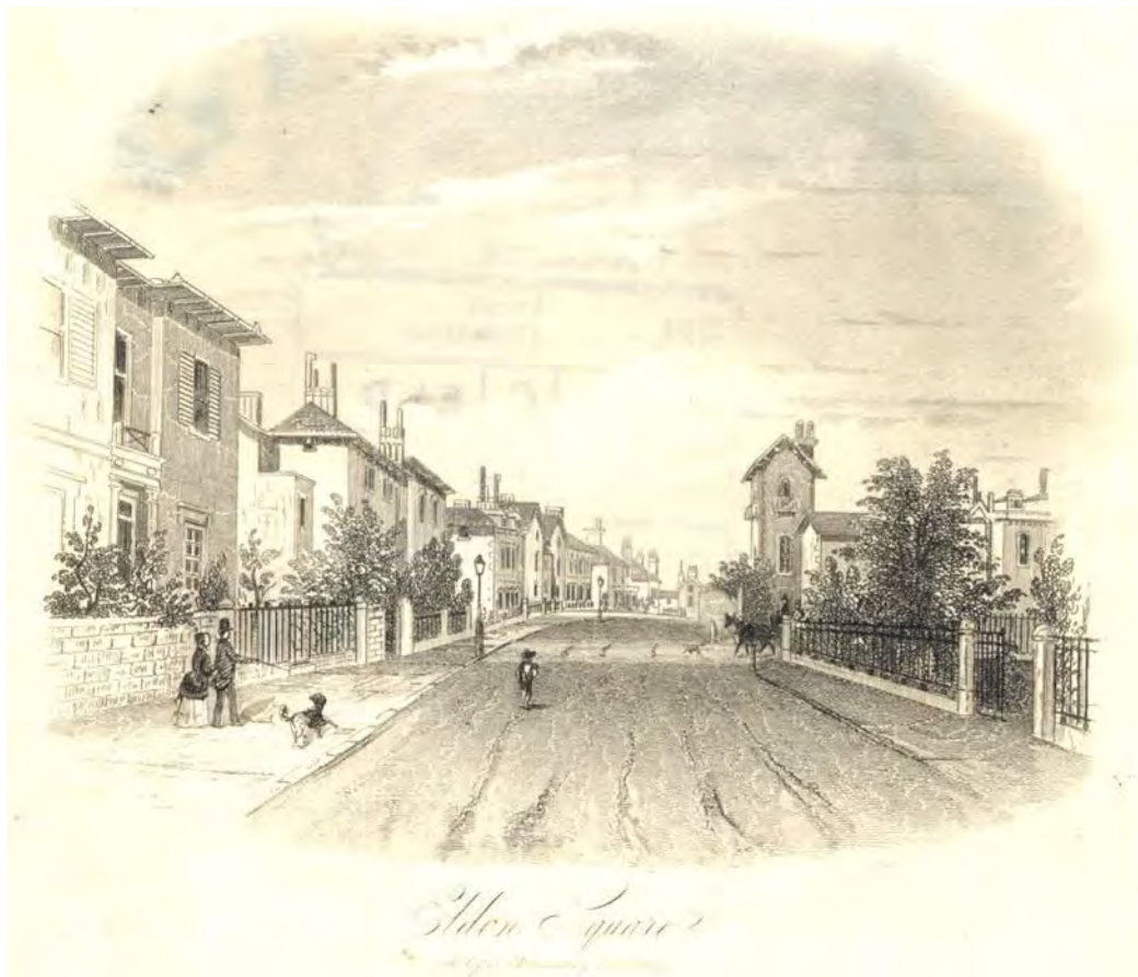
Figure 27: The view north down Eldon road with Eldon House (left) and Eldon Square (right) showing the former three-storey tower of 7 Eldon Square. c1860. Eldon Square a print by J Macaulay courtesy of Reading Library local studies collection
