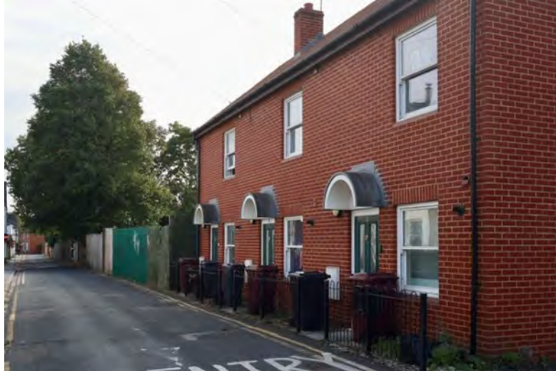
Figure 33: Modern housing on Eldon Terrace (image Zoë Andrews)
