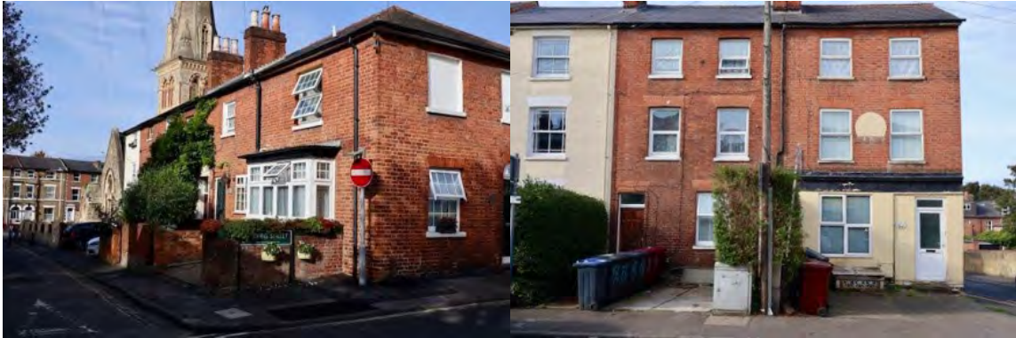
Figure 23: L - former Beehive public house, St Johns Road and R former Golden Lion with Simonds sign painted over, fascia board and shop window bricked in (images Zöe Andrews)
