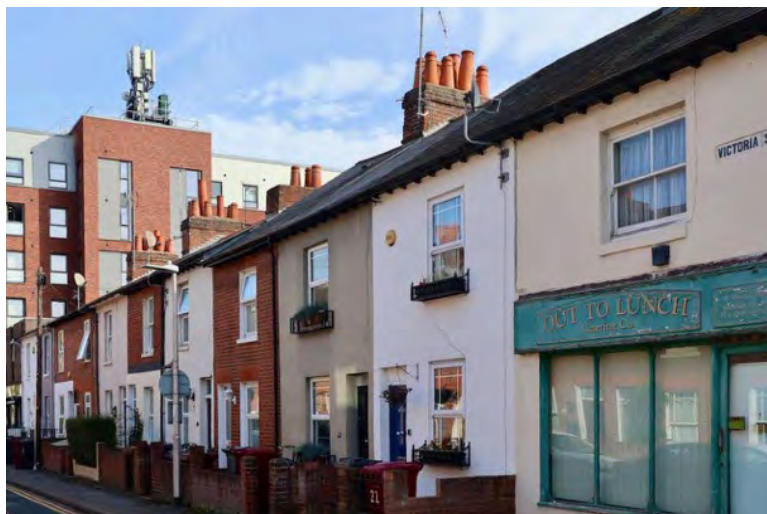
Figure 22: Victoria Street looking north in the direction of Reading College (image Zoë Andrews)
