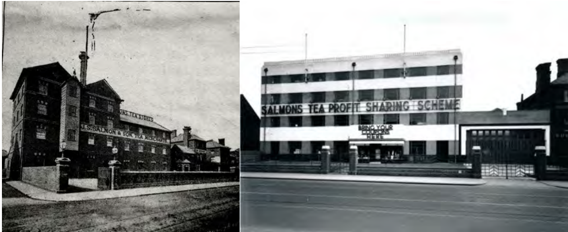
Figure 35: (Left) former Berkshire Brewery while in use as a Salmons tea warehouse c1905 (R W Ford's album 'The Borough of Reading as it Was') and right 1933 the new Salmons tea building on the same site. Images courtesy Reading Borough Libraries Local Studies
